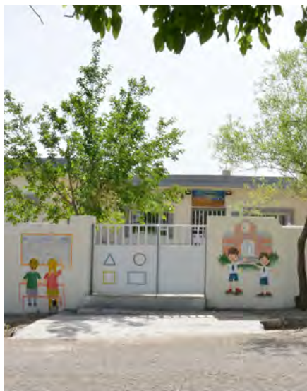
Goshan Primary School Renovation
