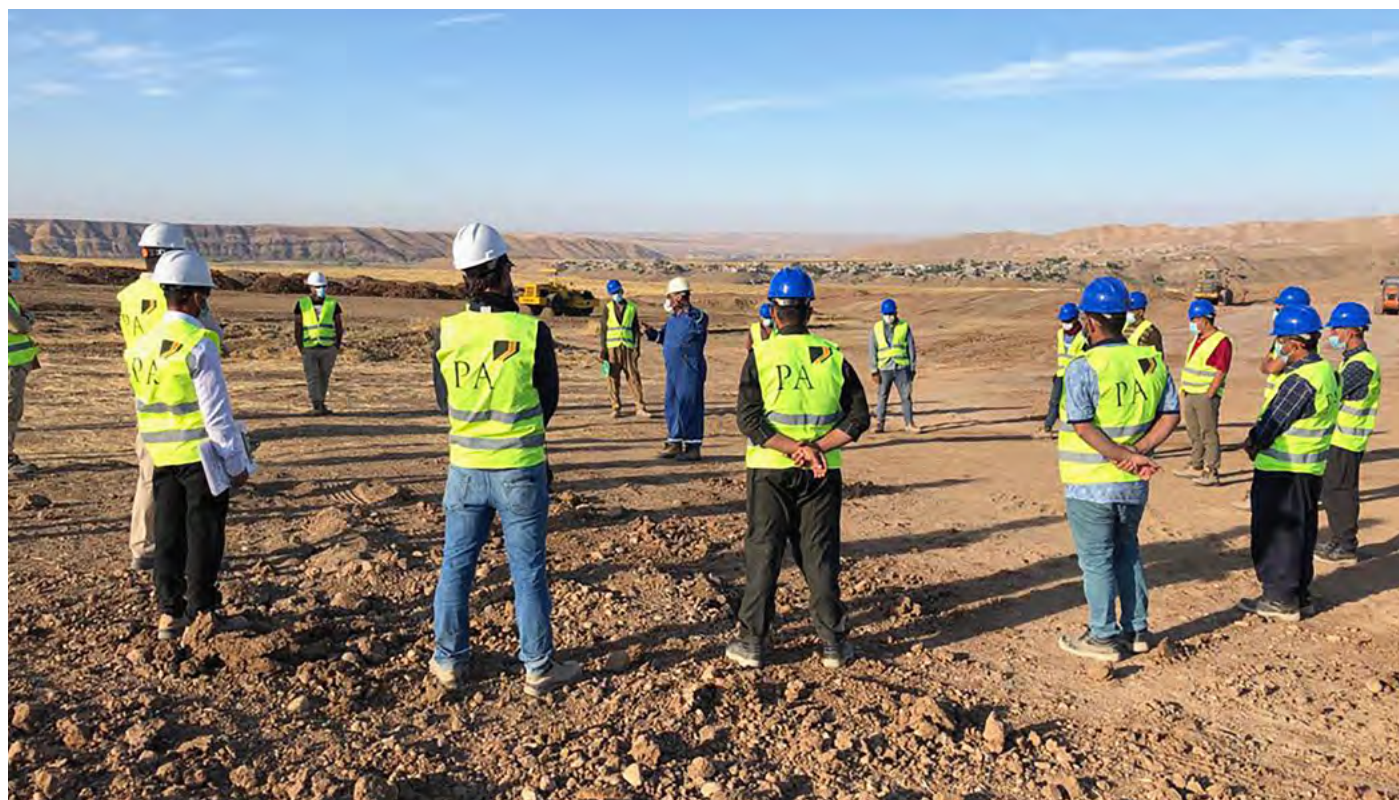
Meetings with contractors during civil construction works at Sarta
