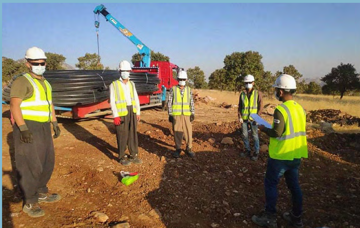
Local company employed by Genel to complete community development project
